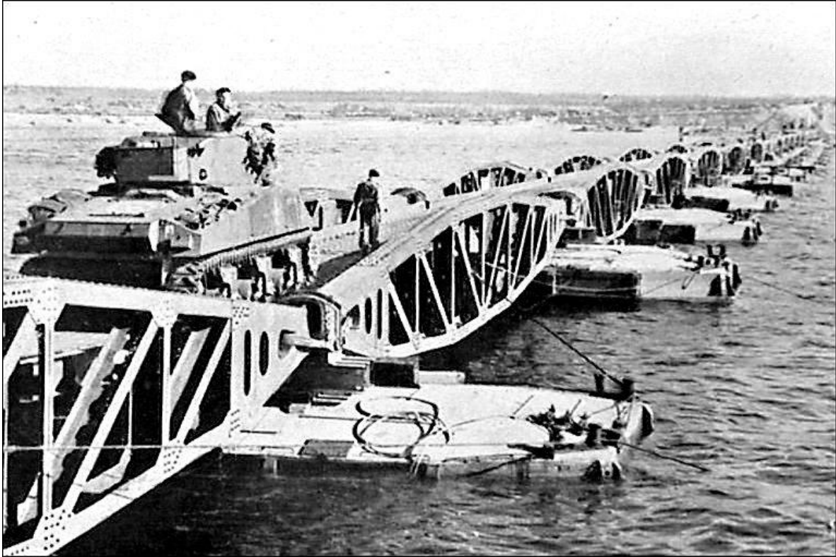
Mulberry “an exceptional piece of engineering and construction”.
